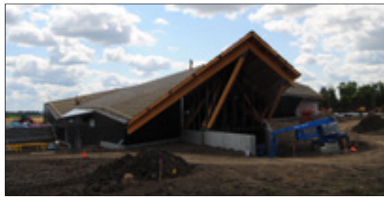
The roof is now covered in clips that will support the metal panels that will cover the building. Keep an eye out for big changes in the roof's look over the coming weeks.
